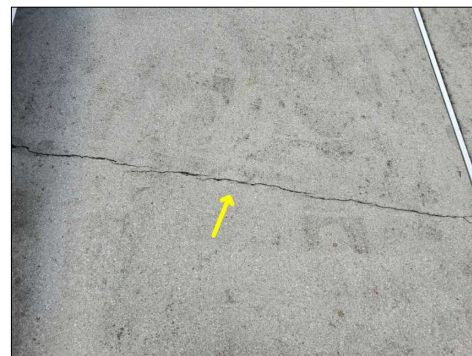
Deck cracking
