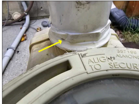
Leaking fitting
