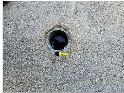
Missing anchor bolts
